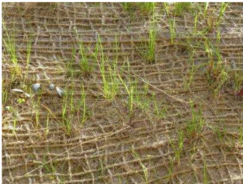
Figure 19: Organic geotextile for erosion control 8
