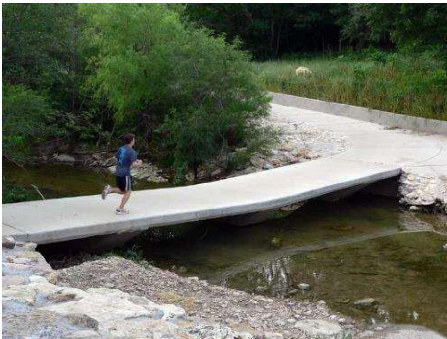
Figure 75: A low water crossing in the US that is not permanently flooded 47
