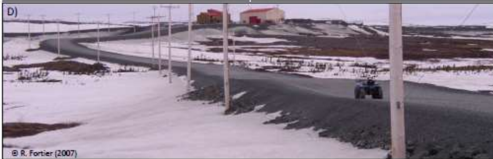
Figure 52: Road in Canada in winter with uneven surface due to frost break
