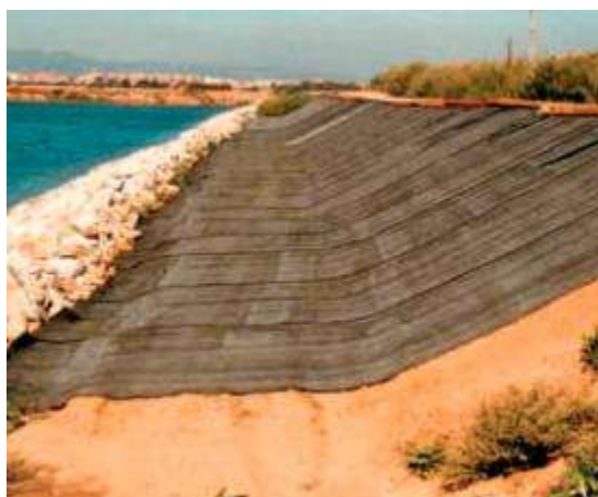
Figure 21: Coastal protection through geotextiles and rocks 10
