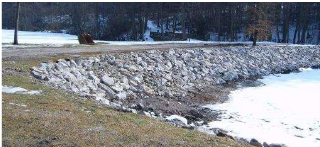
Figure 20: A road at a lake in Bavaria protected by massive rocks 9
