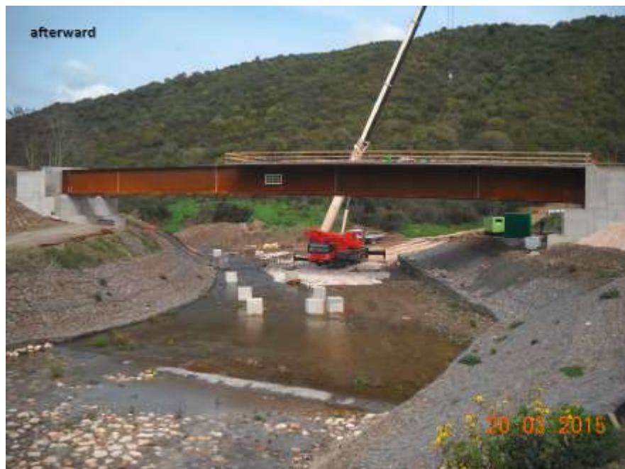
Figure 56: Same location after replacement 34
