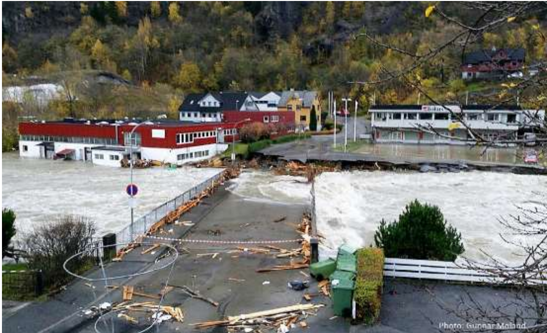
Figure 92: destroyed bridge in Norway due to a flood 62
