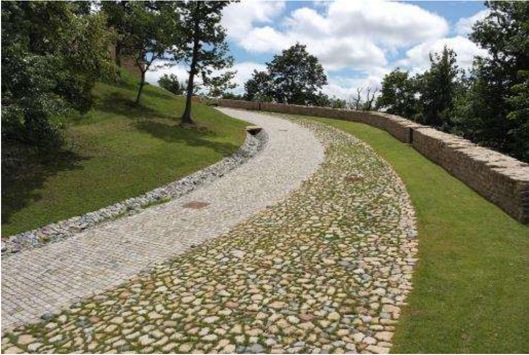
Figure 83: Hard core surface on a historic road in France
