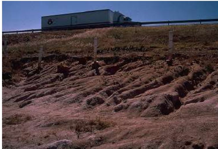
Figure 16: Road embankment damaged by erosion in Canada 5
