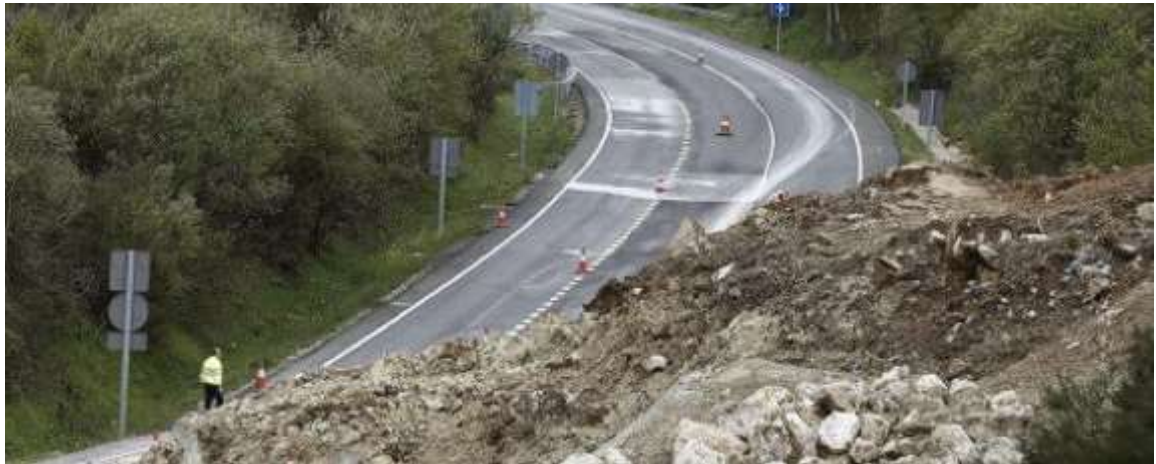
Figure 14: Road in Spain which is completely blocked by a landslide 3
