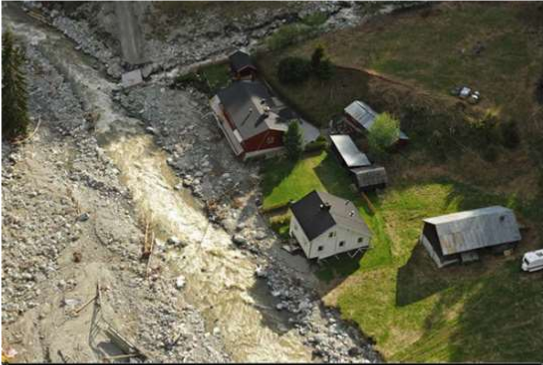
Figure 91: destroyed road and bridge in Norway due to a flooded river with debris 61
