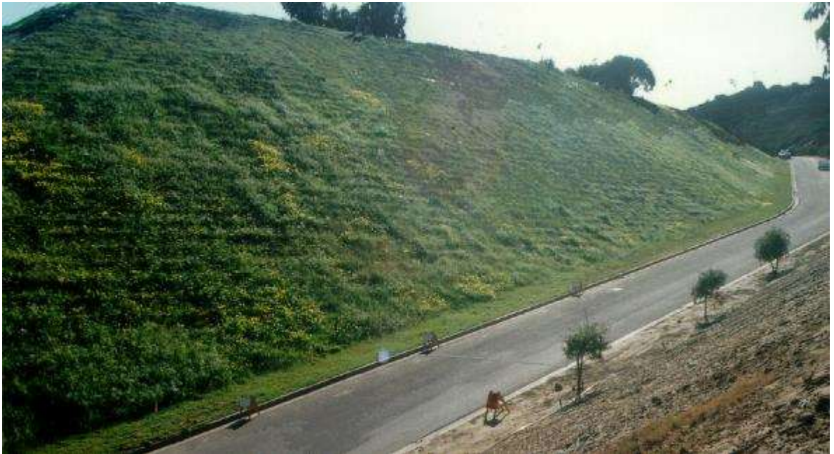
Figure 17: A hill above a small road that got plantation for erosion control 6
