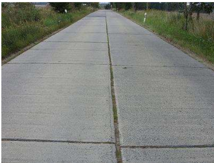
Figure 78:: Rural road with a concrete surface 49
