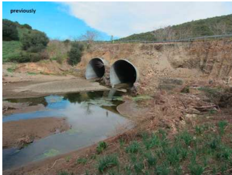
Figure 55: Culvert in a river valley in Sardinia 33
