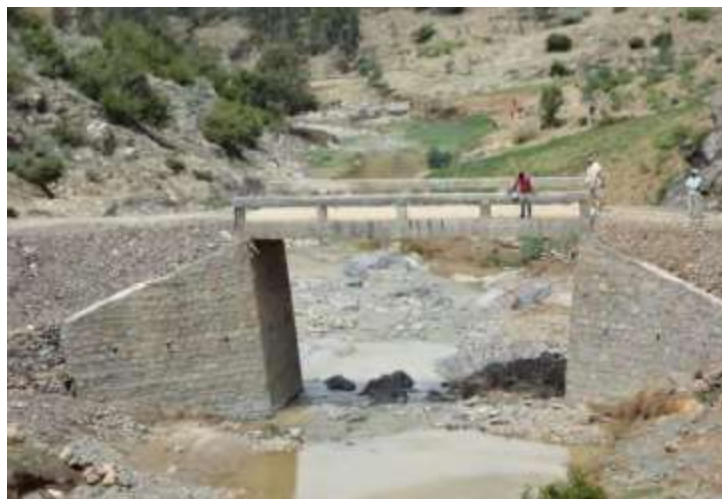
Figure 84: Bridge in Ethiopia that is guaranteeing road access during wet season
