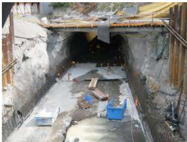
Figure 94: Railway plan for Varbergs tunnel in south of Sweden (construction 2019-2024) M Baumann
