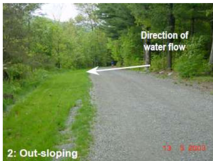
Figure 103: Cross slope of a road where both lanes are inclined towards the same direction 67
