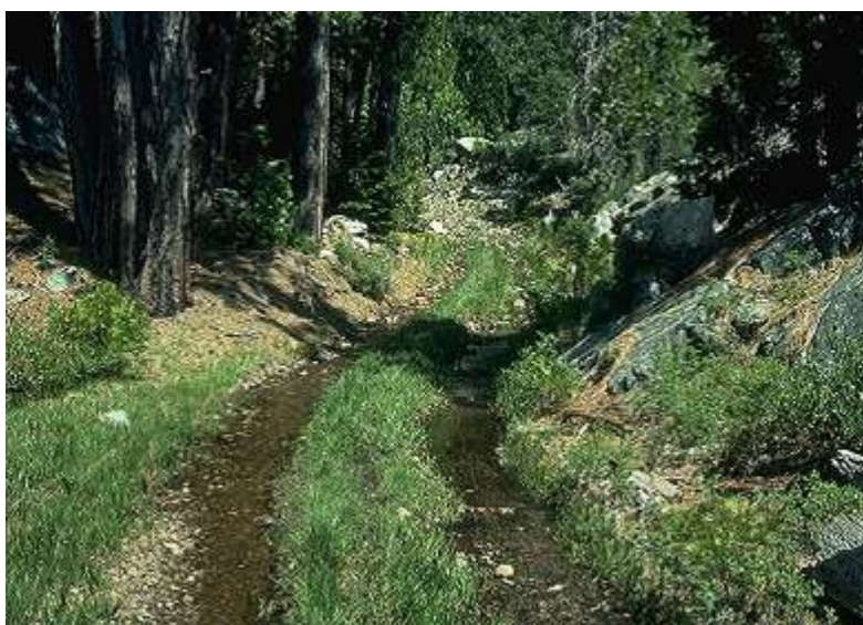
Figure 96: rural road in the USA that turned into a streambed 71
