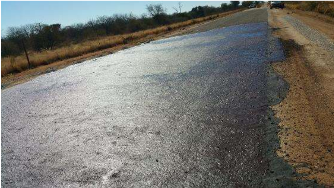
Figure 86: Cape Seal on a gravel road in South Africa 56
