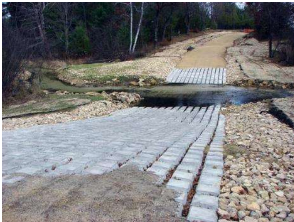
Figure 74: Low water crossing designed and built by the US army 46
