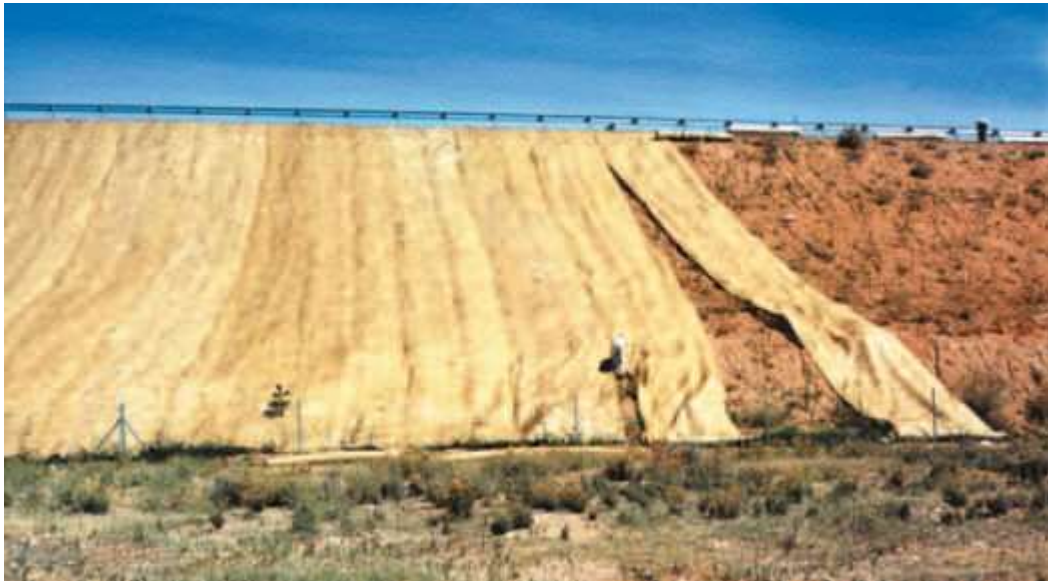
Figure 18: Geotextiles are getting installed at a road embankment 7
