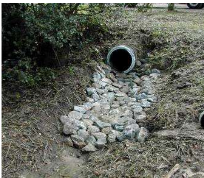
Figure 70: Discharge of a culvert on armoured underground 42
