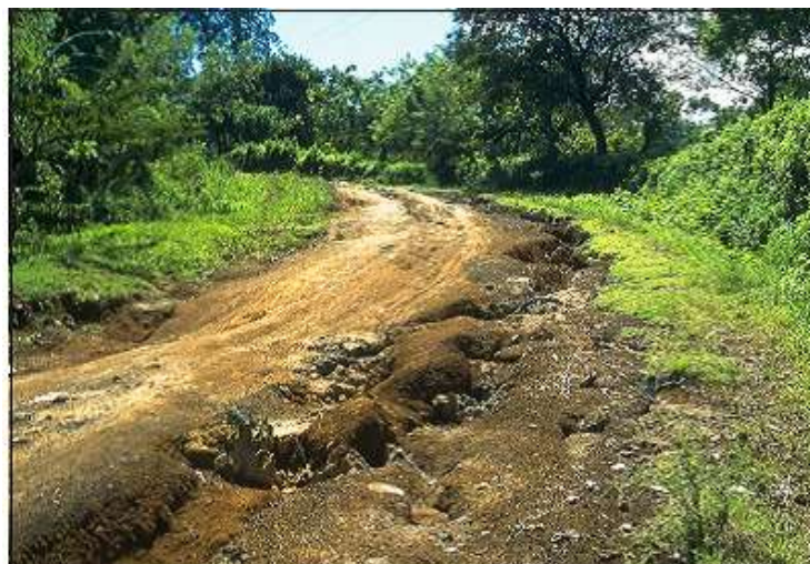
Figure 95: road in Central America damaged by erosion 68
